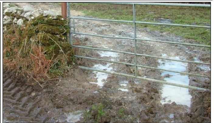
Built in wet weather, needs finishing with chip.
