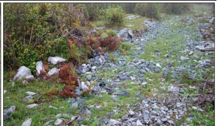
Surfaced with large chip, difficult for stock to use.
