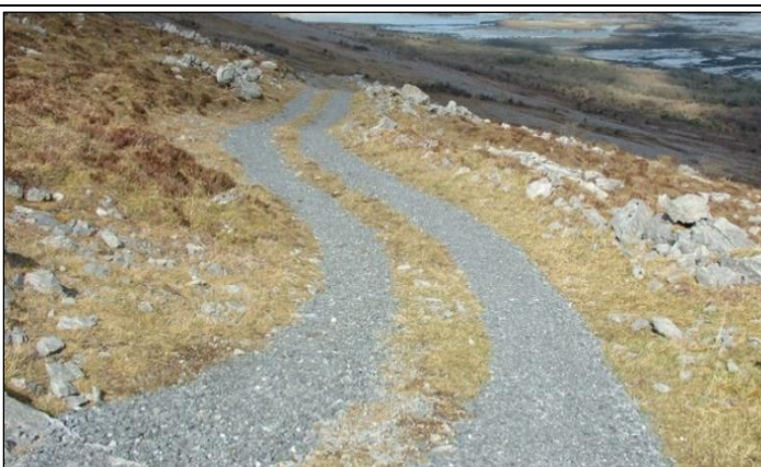
Existing track, with newly surfaced wheelings.
